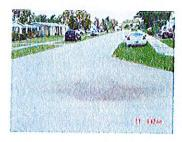
Poorly graded/settled asphalt and pavement. Many areas that flooding and ponding were observed showed signs of poorly grading asphalt that did not allow proper flow of stormwater to the catch basins. Other locations showed signs of settling asphalt. This may create low points on roads and driveways that could pond.
