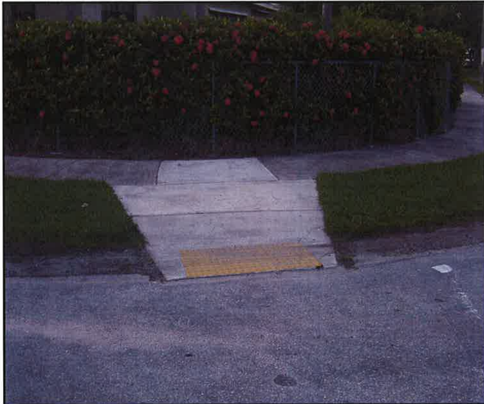
Picture 1: Corner with ADA accessibility
