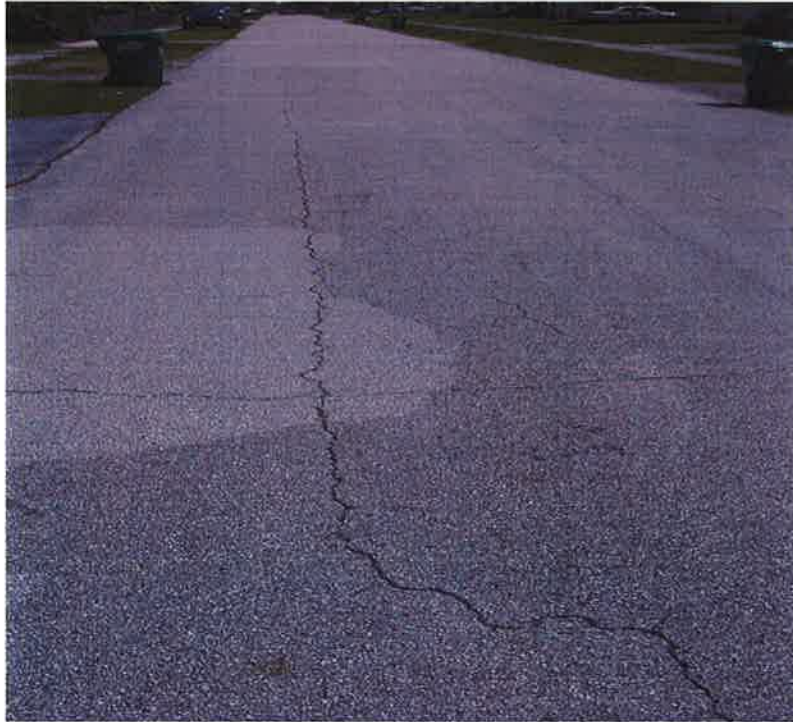
Picture 12: Longitudinal Cracks
