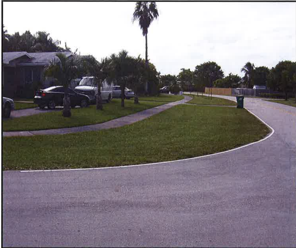
Picture 2: Corner lacking ADA accessibility
