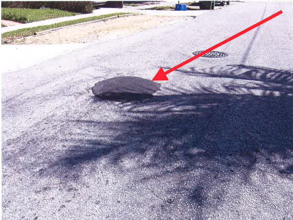
Picture 10: Repaired Pot Hole
